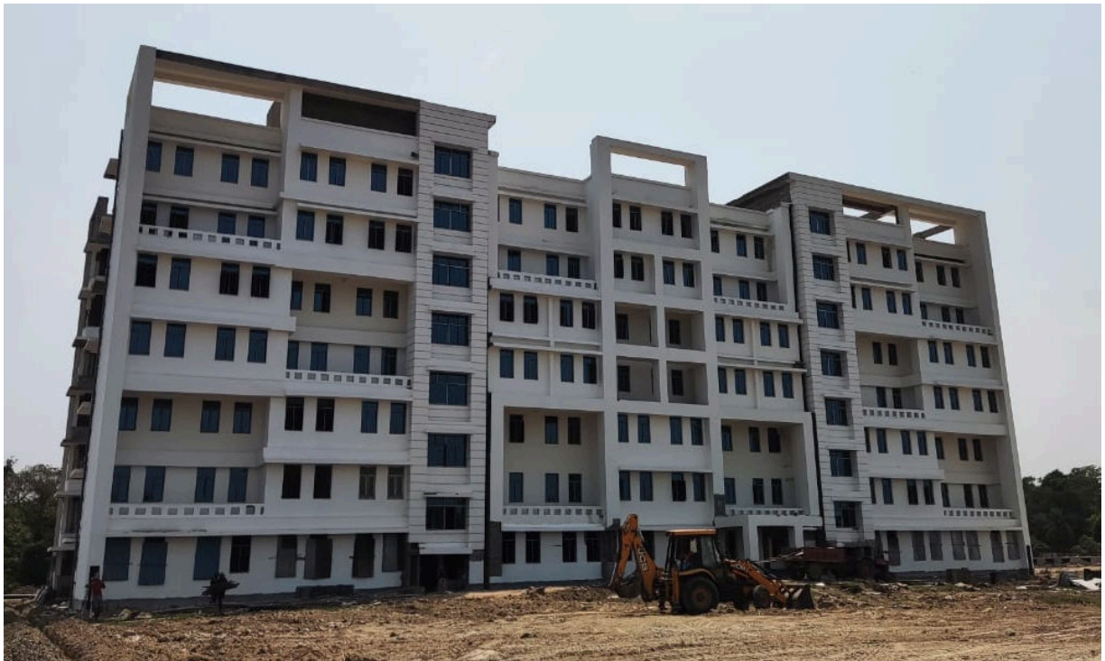
Boys' Hostel (Under Construction)
