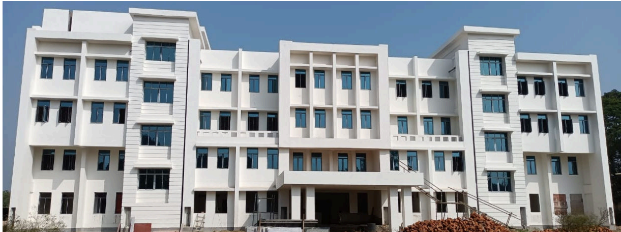
Girls' Hostel (Under Construction)
