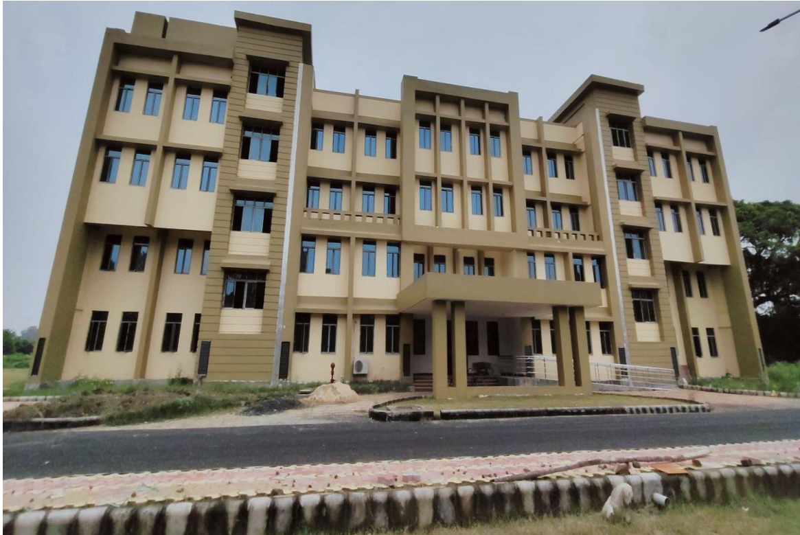
Girls' Hostel (under construction)
