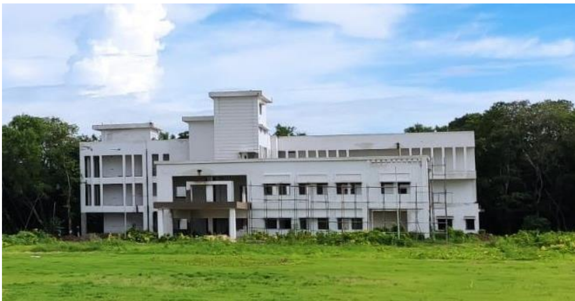
Guest House (under construction)
