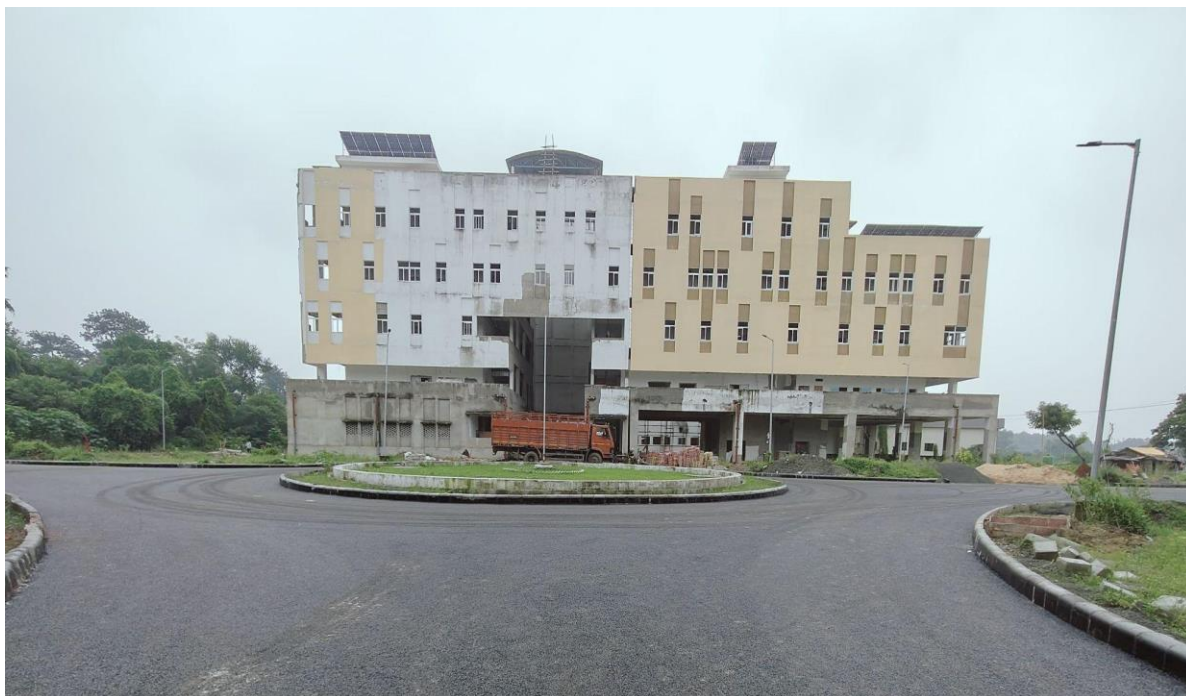
Administrative Block (Under Construction)
