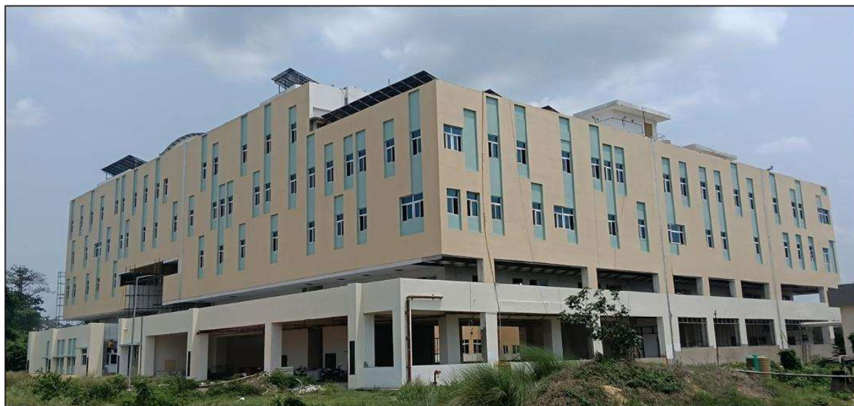
Administrative Block (3D view, Under Construction)
