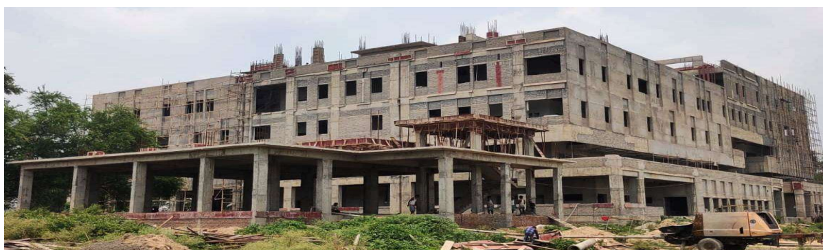
Photograph: Administrative Block(under construction)
