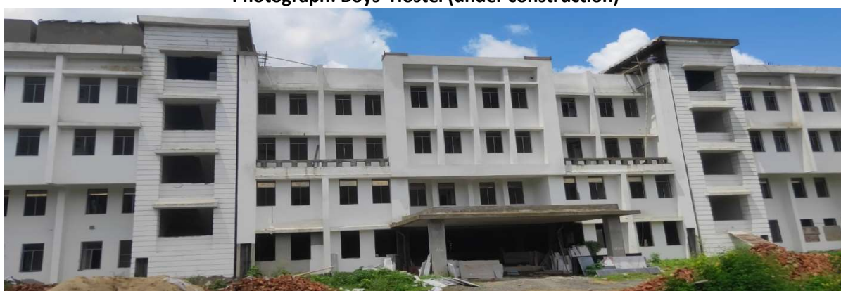
Photograph: Girls' Hostel (under construction)
