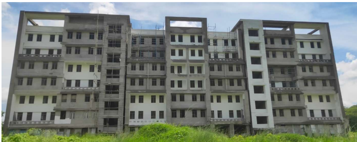
Photograph: Boys' Hostel (under construction)
